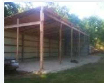
"I used treated telephone poles which I acquired from a friend to create 6"x6" beams for the supports, and 2"x4" boards for the roofing. I saved a lot of money using salvaged lumber and
