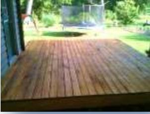
“I created the deck using telephone poles as a base, the framing boards underneath were from a red oak tree that I milled, and the top boards are white oak. It was really easy to make.”
